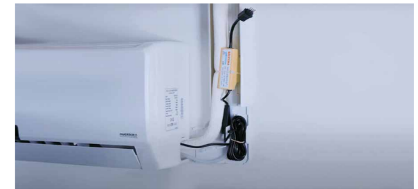
Solution with an externally incorporated condensate pump.
